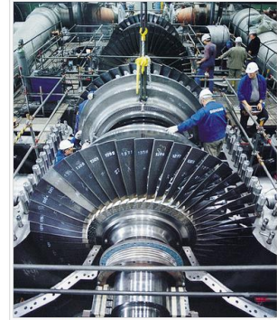
A steam turbine with the case opened. Most electricity is produced by thermal power stations with turbines like this one. Electricity consumption and living standards are highly correlated. [1] Electrification was voted the most important engineering achievement of the 20th century. [2]
